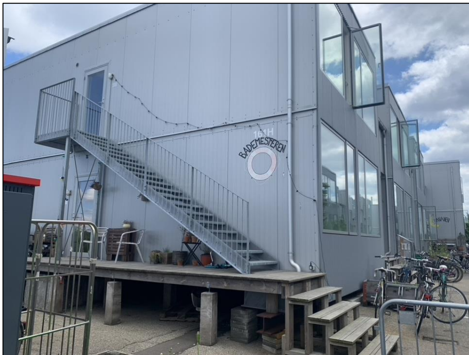
Figure 11: Another picture of the shipment container apartments and more bikes can be seen. There is also no foundation as a base to the apartments.
